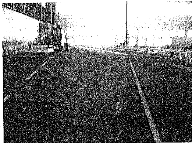
CARRIER DECK FOR TRAINING SAILORS IN FLIGHT DECK OPERATIONS. DECK IS ABOUT 12 FEET ABOVE THE FLOOR OF THE HANGAR.
